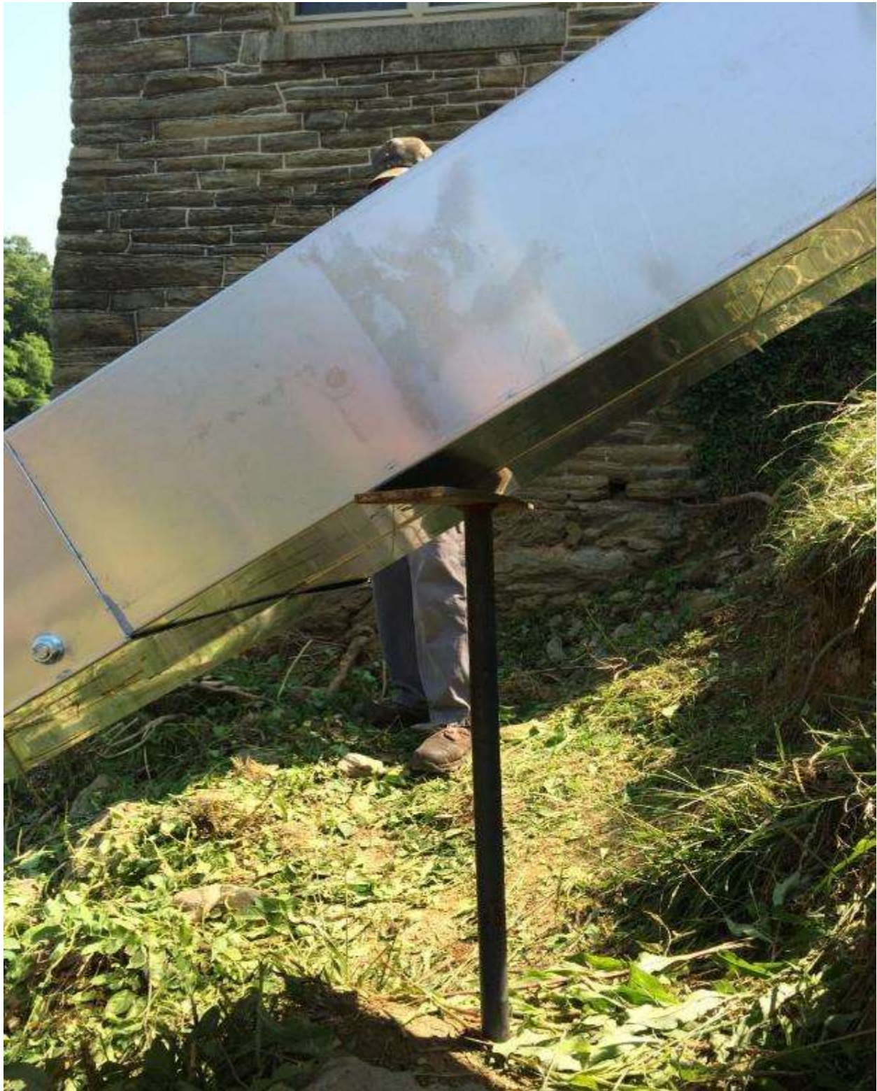
Figure 3.1-2: T-Bar Support for Ramp Support, Octoraro Creek
