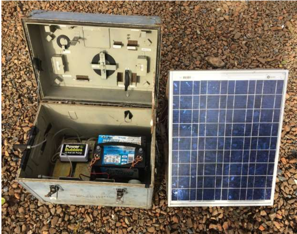
Figure 3.1-7: Aerator Powered by a Marine Battery and Charged by a Solar Panel, Octoraro Creek
