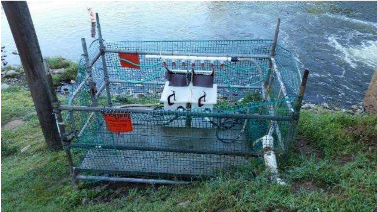
Figure 3.1-4: Manifold for Garden Hose Supply Lines for Attraction Flows, Octoraro Creek
