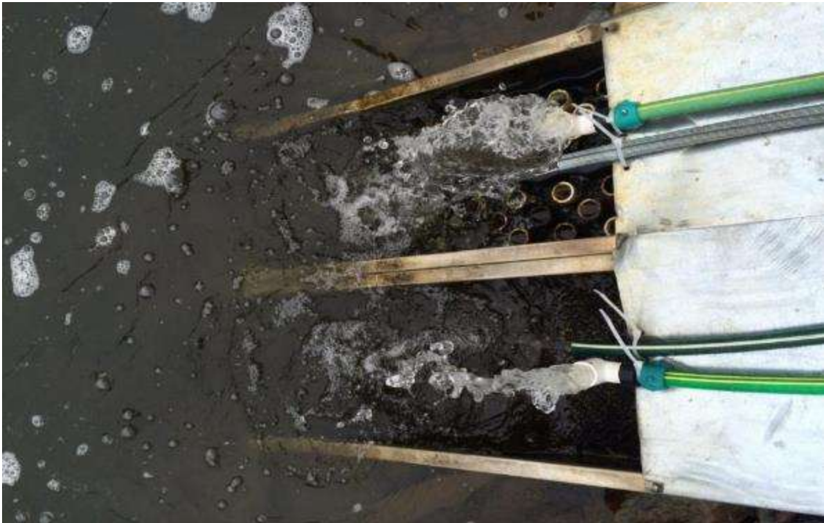
Figure 3.1-3: Additional Attraction Flow Hose Added to Entrance, Octoraro Creek
