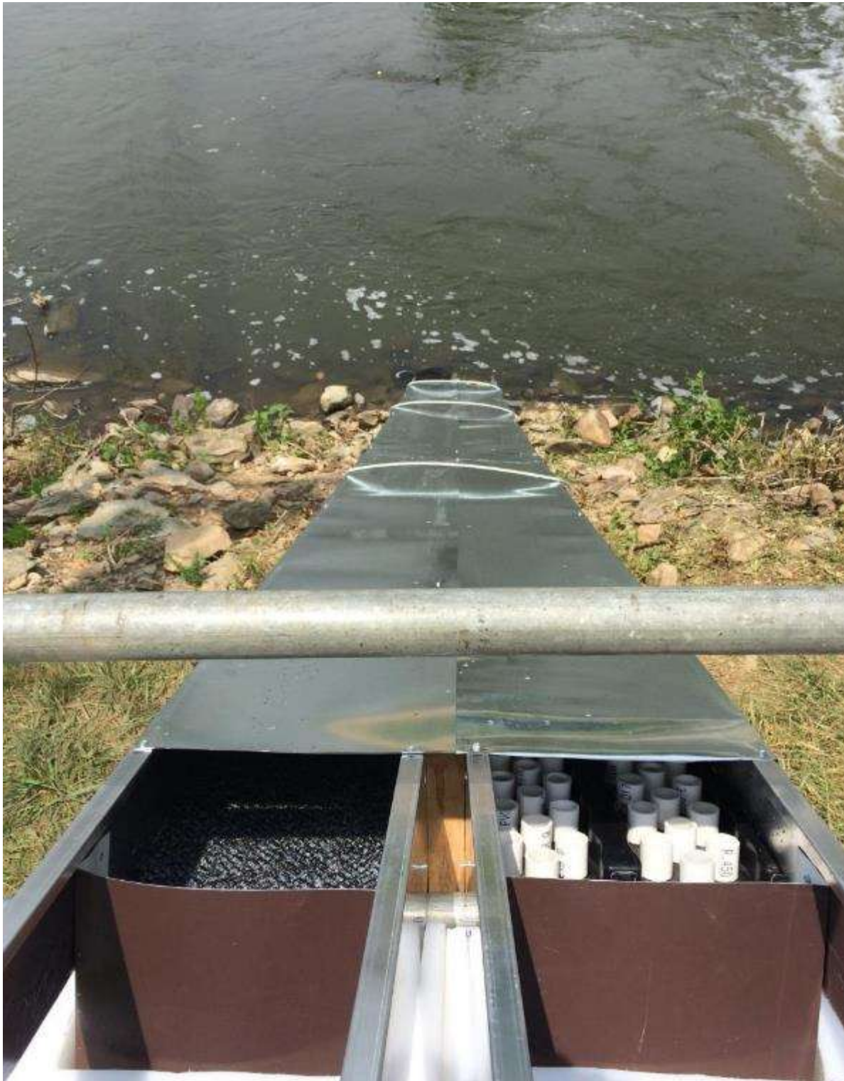
Figure 3.1-1: Photo of Enkamat and Milieu Substrate Installed in Ramps, Octoraro Creek
